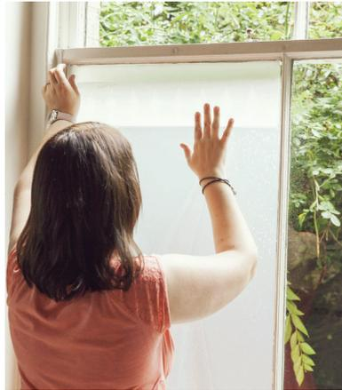
Take the film to the window making sure you keep it taut, allow the film to flow onto the glass and slide into position
