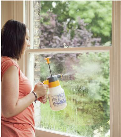
Before beginning installation, ensure your glass is as clean as possible. Next spray the entire pane with the soapy water before applying the film
