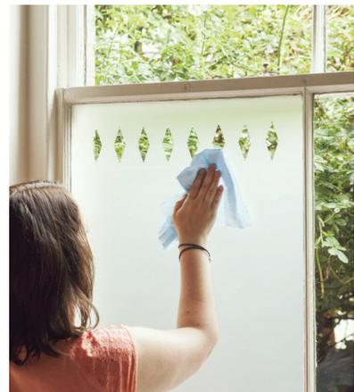
Finally wipe off any remaining water from the film and the frame being especially careful around the edges of any cut outs not to lift the film
