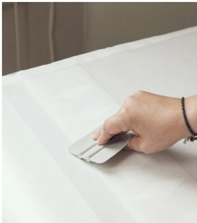
Card over the design using the Squeegee supplied to increase the bond between the application tape and Frostbrite film
