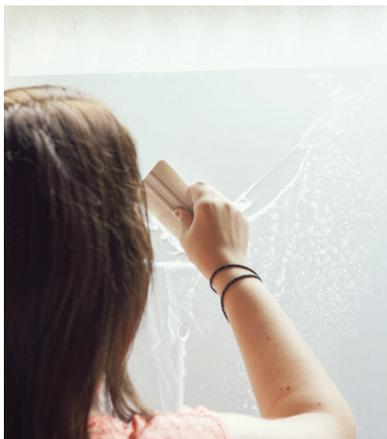
Work from the top pushing any bubbles out to the edges, whilst ensuring the film doesn't move, you can repeat this process again to ensure all water is removed. Then leave to dry for 24 hours
